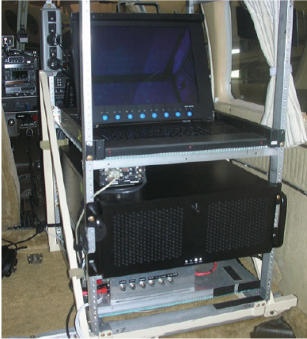
Figure 5. Rack Unit Installation
